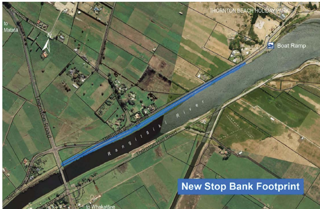
Fig 4: Lower Rangitāiki stopbank upgrade works remaining - left bank
