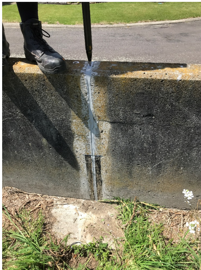
Photo 1: Expansion joint repair - Landing Road floodwall
