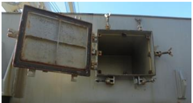
Natural vents with grill removed & door open.
