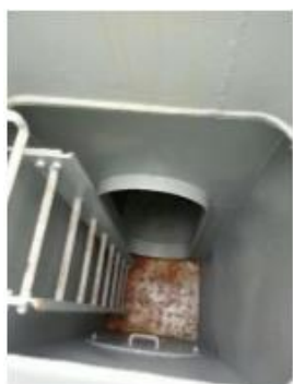
Dog-leg preventing correct pallet fumigation
