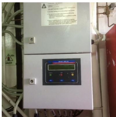
Smoke Detection Unit in CO2 Room
