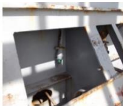
Drains at the side, seal up now
