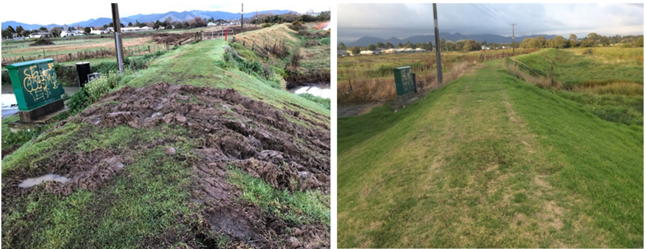
Photo 4 and 5: Stopbank damage at Tarawa Creek outlet (before and after)
