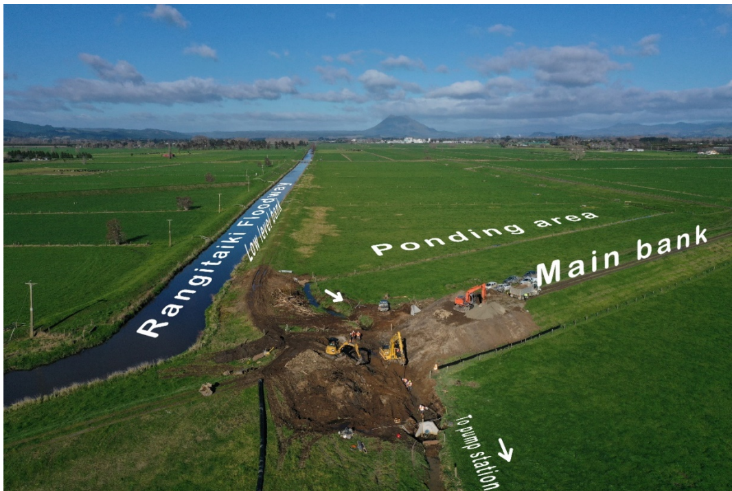
Fig 3: Stage 6a preparatory culvert works
