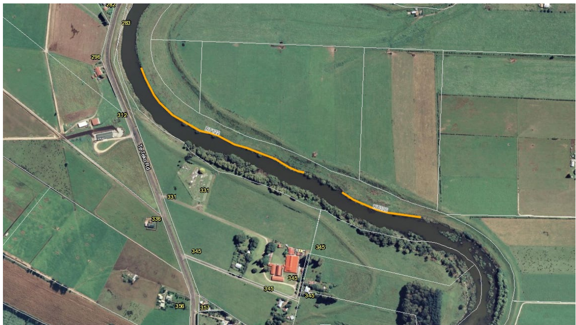
Photo 1: RT122 and RT336 locations
