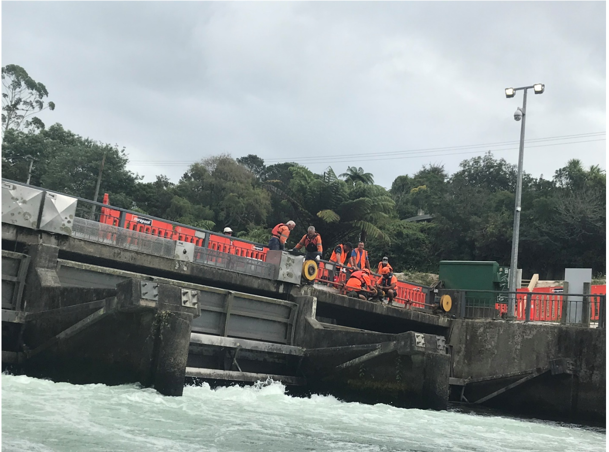
Figure 1 Okere Gates – BOPRC Rivers and Drainage staff and contractors removing radial gate for scheduled maintenance – March 2020.
