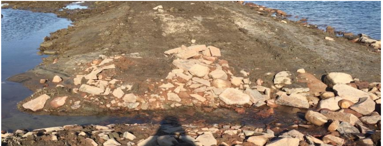
Photo 3: Water flows over the rocks between the river on the right of the photograph and the constructed wetland on the left; plants will be added to create shade. (Reids Canal bifurcation wetland, Thornton).
