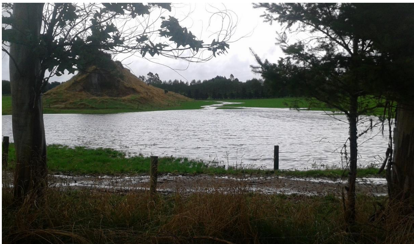
Figure 29 A storm water run-off event filling a Detainment Bund PS120 ponding area located on prime pasture. (Photo J. Paterson)
