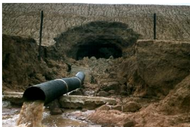
Figure 33 An example of ‘piping’ erosion. Poor pipe haunching, inadequate compaction around the pipe during installation, causing embankment failure. (Pipe cross section diagram and photo from FEMA 2005).
