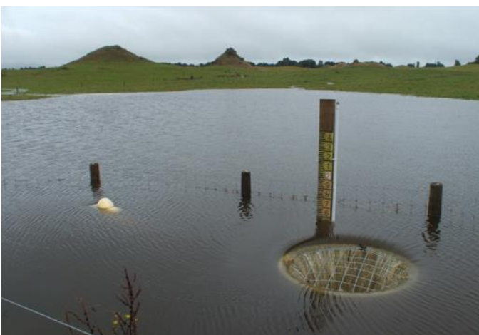
Figure 6 (left) DB full and skimming off overflow. (Photo D. Clarke) (right) DB empty, and growing grass, its usual state. (Photo J. Paterson)
