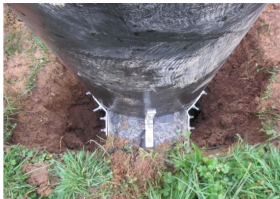
(b) Rear view – pipe/riser joint.
