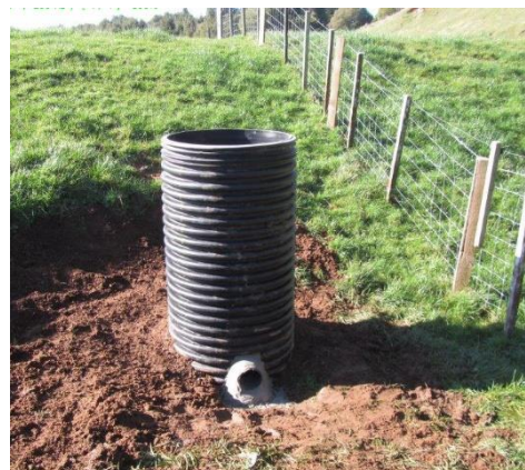
Figure 18 Contrasting design features of a Detainment Dam outlet (left) and a Detainment Bund PS120 outlet fitted with an Upstand Riser (right). Both are pictured at time of installation, hence the disturbed soil. Note the new embankment structures in the background are well established in pasture.
