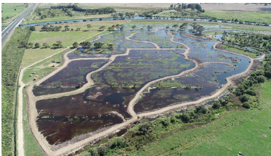
Figure 6: Tumu Kawa land photographed on 1 May 2020, after construction
