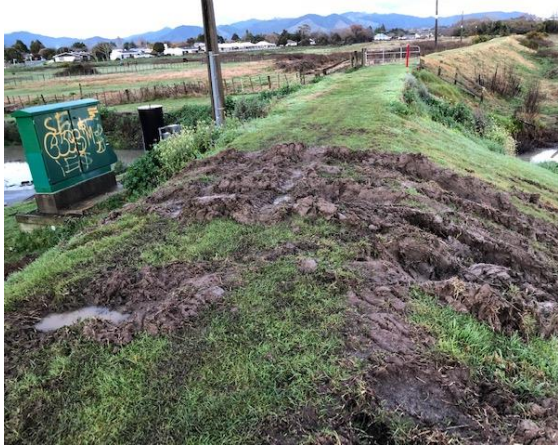
Photo 2 and 3 - Stopbank damage at Tarawa Creek outlet (before and after)
