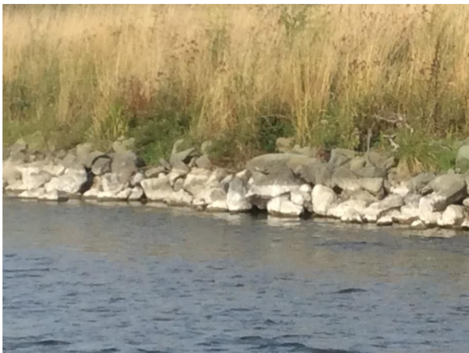
Photo 10 - Ernest rock works – note vegetation growth and gaps in rock (eel habitats)
