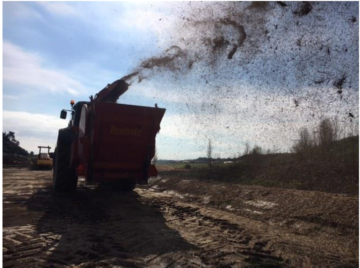
Figure 4: A hay mulcher spreading mulch to stabilise the earthworks site at the Tauriko Business Estate development
