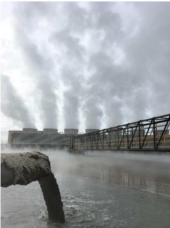
Figure 5: Looking across a clarifier, which is used to treat wastewater from the paper and pulp production process at the Norske Skog Tasman Ltd plant in Kawerau
