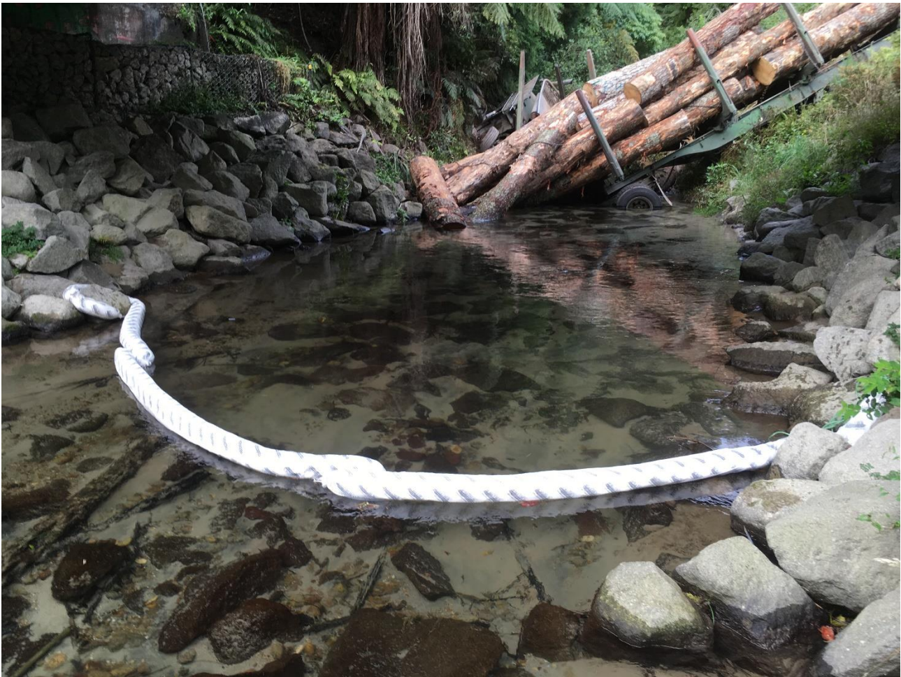
Figure 8: Staff deploy booms in the Tautau Stream to capture debris and hydrocarbons, following traffic incident in March 2019
