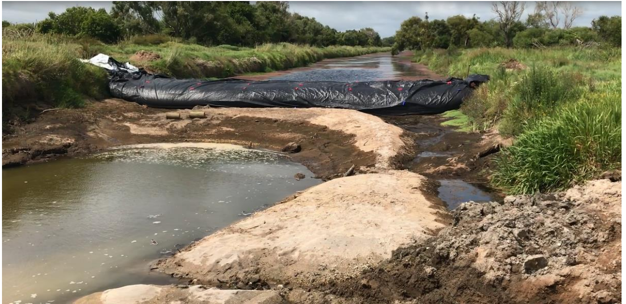
Photo 6: Canal 109 temporary dam
