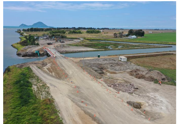
Photo 2: View north showing the bifurcation cut February 2020
