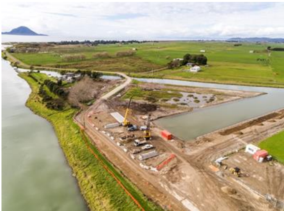
Photo 1: View north showing the bifurcation cut September 2019
