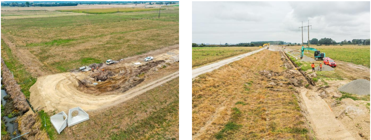
Photo 5: Stage 7 works February 2020
