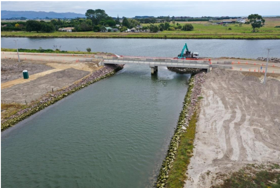
Photo 3: Bifurcation cut and new bridge
