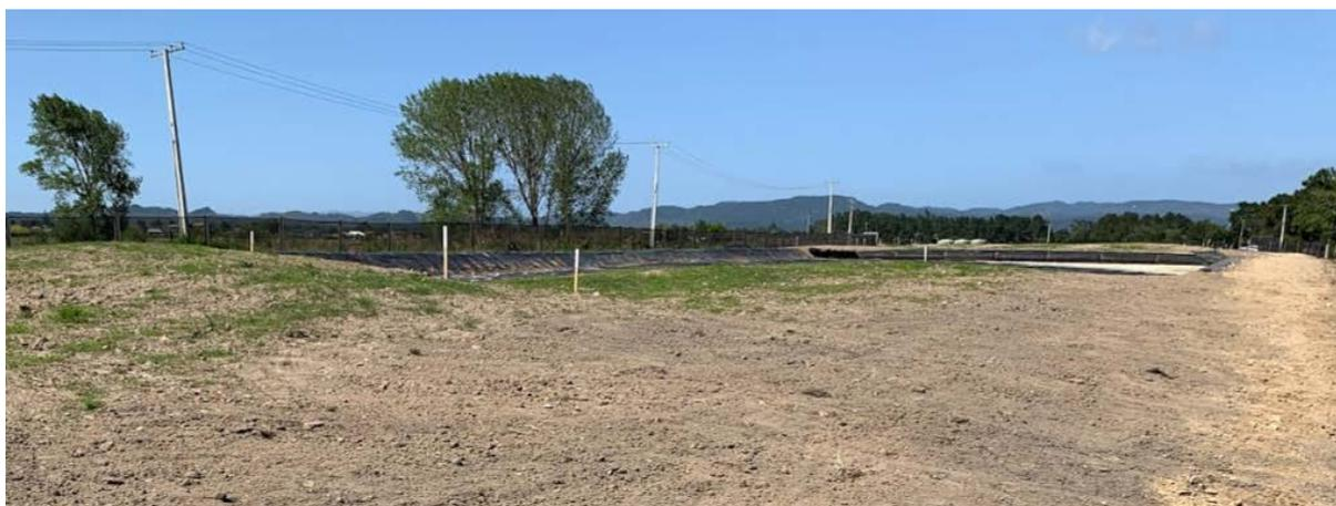
Figure 4. Completed topsoil capping at CS3.
