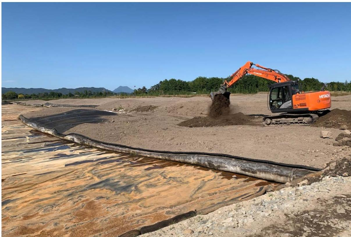
Figure 2. Topsoil capping at CS1 nearing completion.
