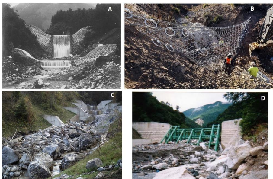
Fig. 2 Debris-flow structures. A: Masonry dam. B: Ring-net. C: Check-dams. D: Grill.
