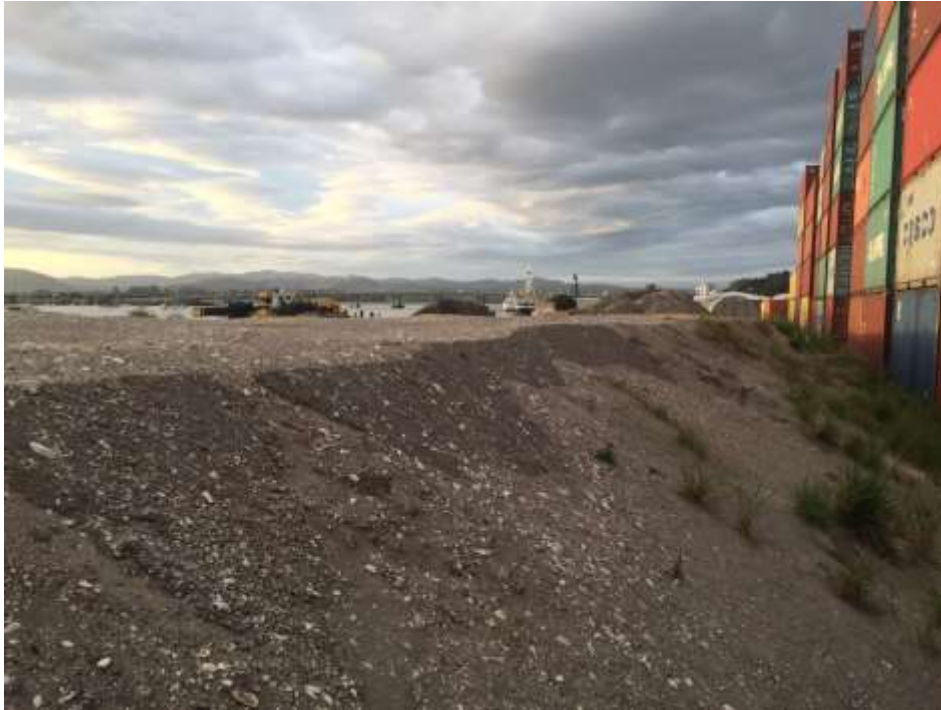
Photo 18 Thin polymer applied to dredging sand stockpiles [Sulphur Point, 6:45 AM 21 Oct 2016]
