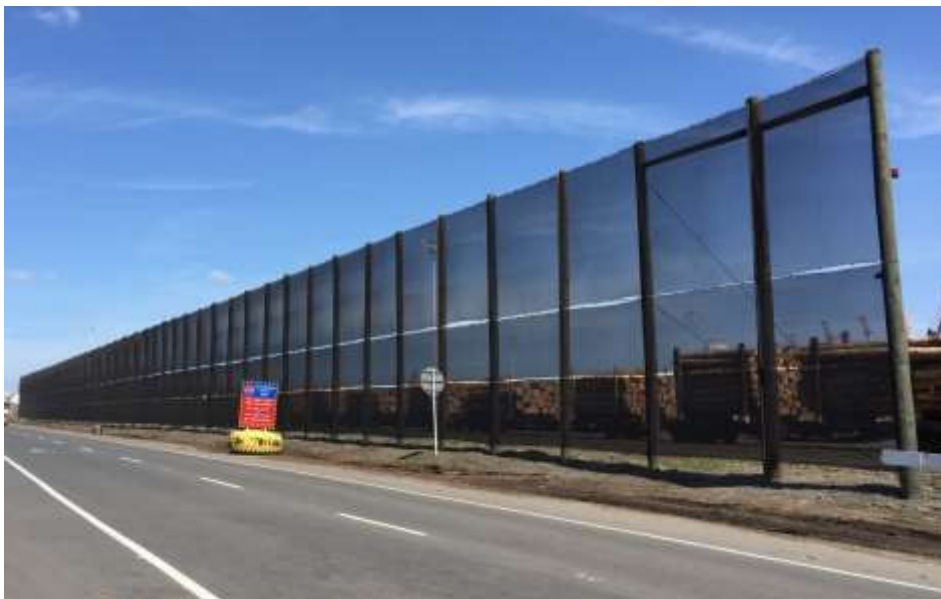
Photo 8 Wind break fence on eastern side of log handling area. [Tasman Quay, Mt Maunganui Wharves 11:48 AM 18 Oct 2016]
