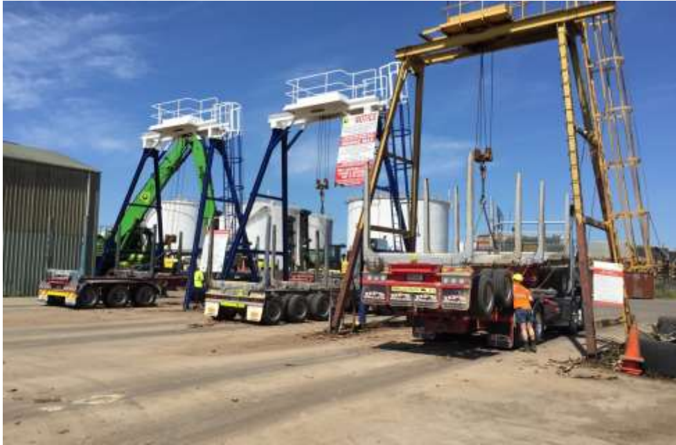
Photo 16 Truck debarking area [Mt Maunganui Wharves 1:23 PM 17 Oct 2016]
