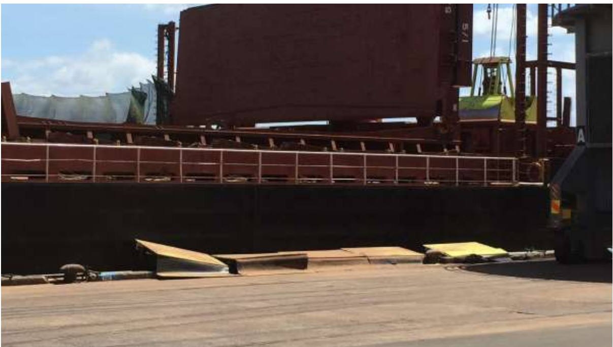
Photo 21 Save-all (metal) under path of crane grab during unloading of palm kernel. [Sen Treasure, Mt Maunganui Wharves, 12:44 PM 17 Oct 2016]
