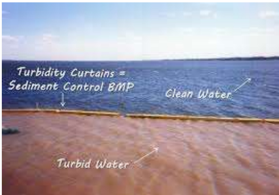
Figure 9 Example of silt screen
