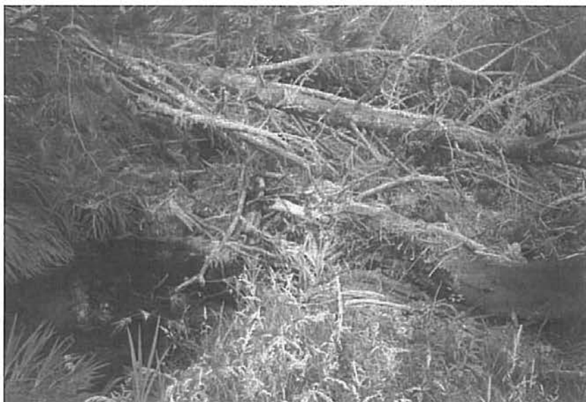
Figure 11.3 The second debris dam, low flows pass through the blockage.
