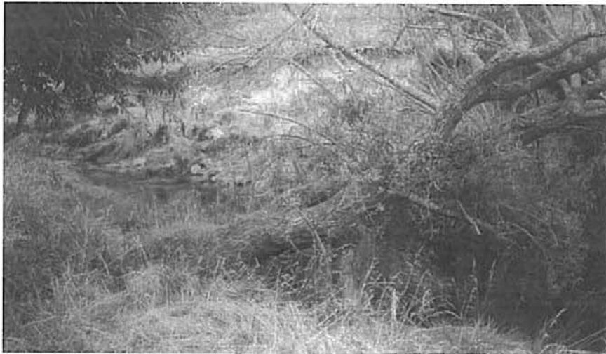
Figure 12.6 Typical potential tree blockage at 1km above SH2, while extensive erosion is evident in the background.
