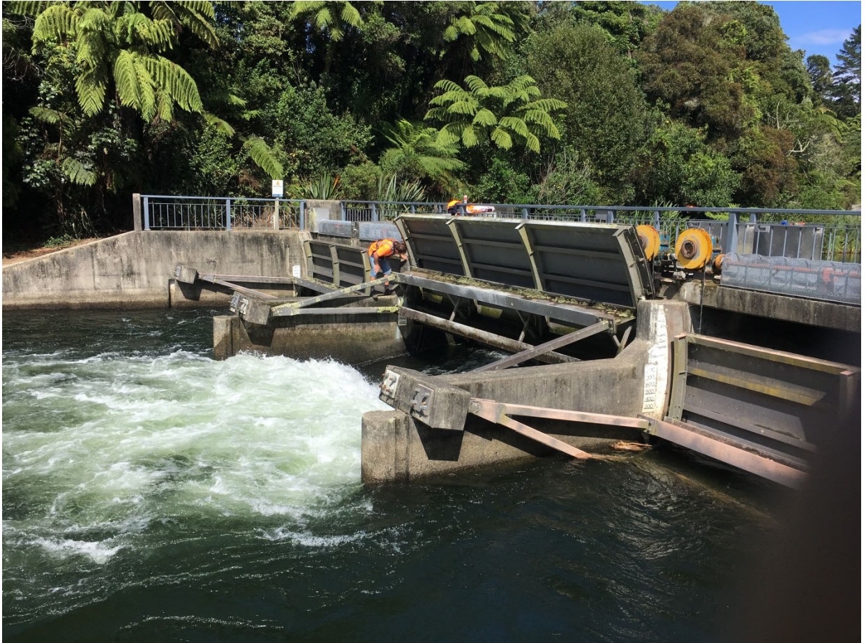
Figure 1 Okere Gates – Technicians calibrating the Okere Gates following replacement of the main lifting ropes – April 2019.
