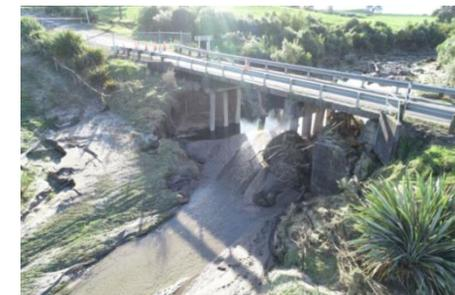
Rerewhakaaitu Bridge – severely damaged as a result of the April 2018 flooding
