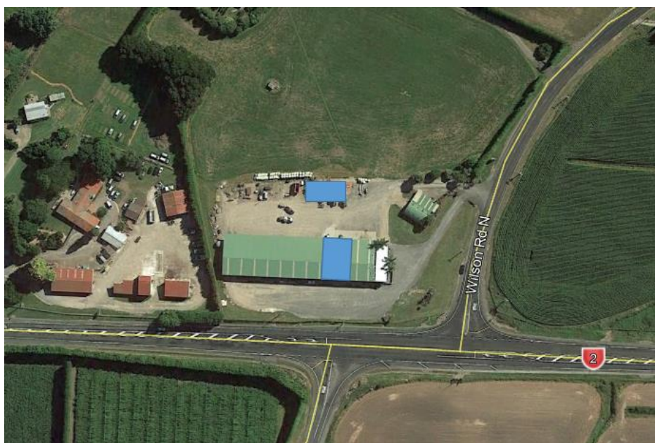
Fig 1: Kaituna Depot location
