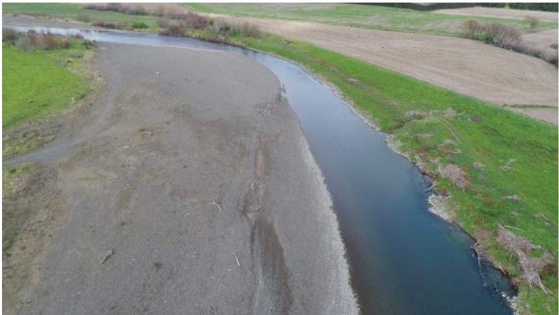
Photo 7: Rewa Hill overflow diversion required
