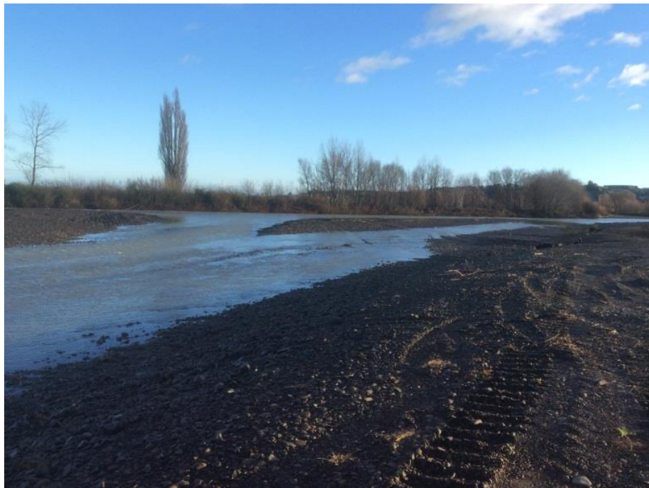
Photo 3: Carters overflow channel
