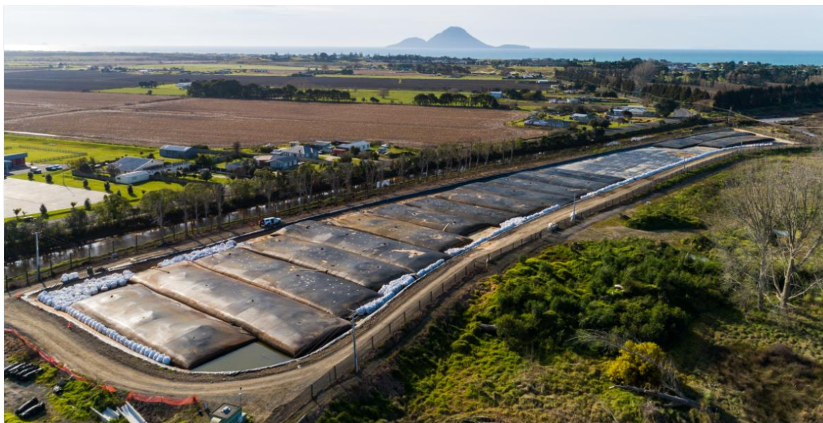
Figure 2. Geotube bags filled at CS3
