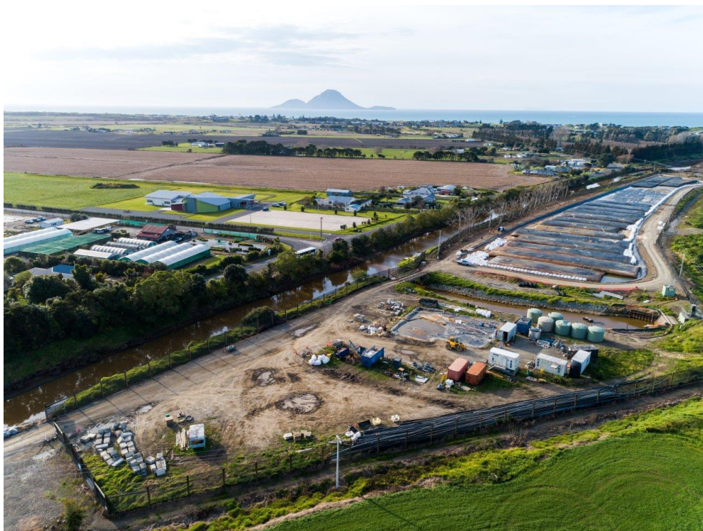
Figure 4. Ongoing clean-up of Containment Site 3.
