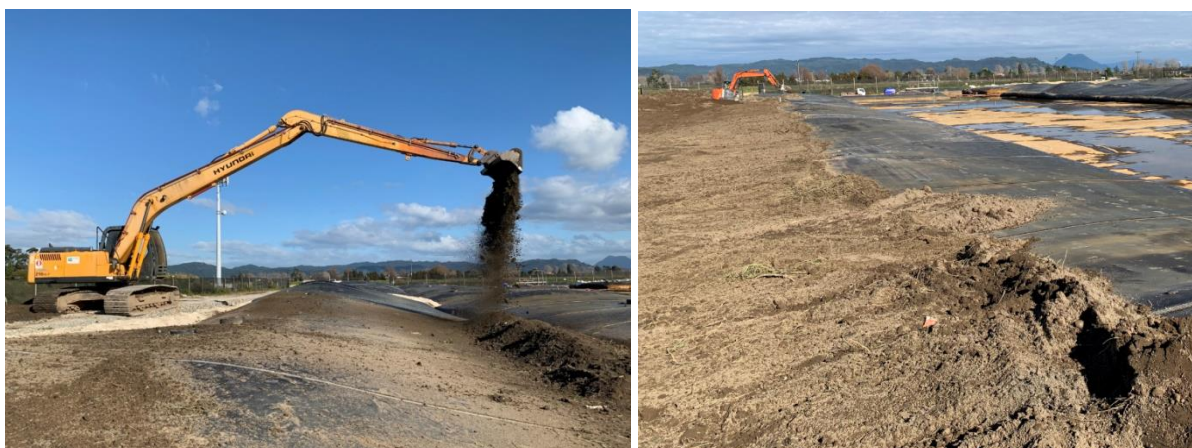
Figure 5. Topsoil capping at CS1.
