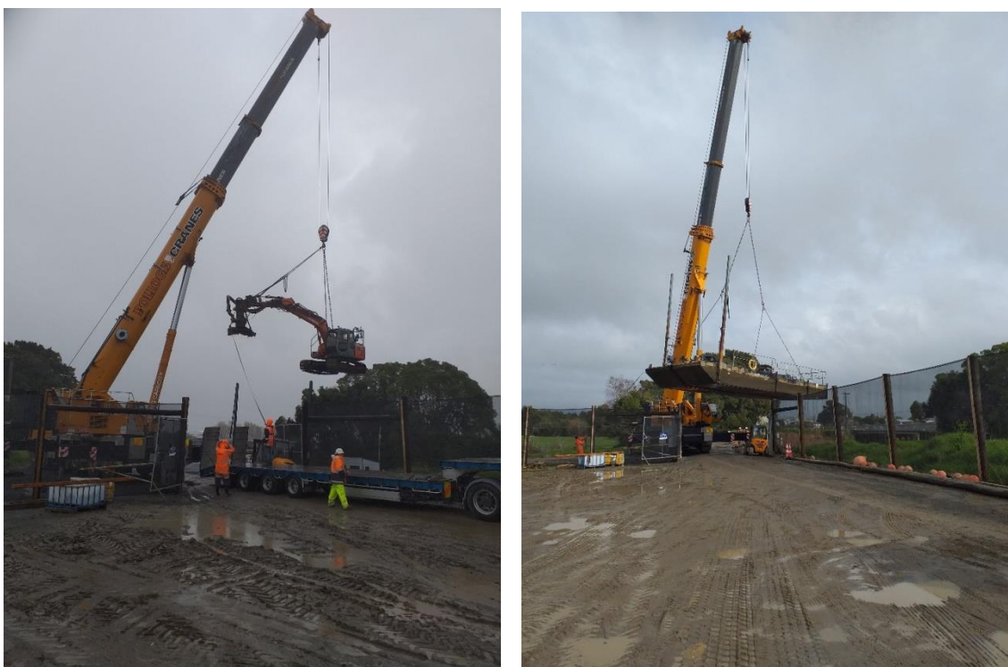
Figure 3. Demobilisation of the dredging excavator and barge.
