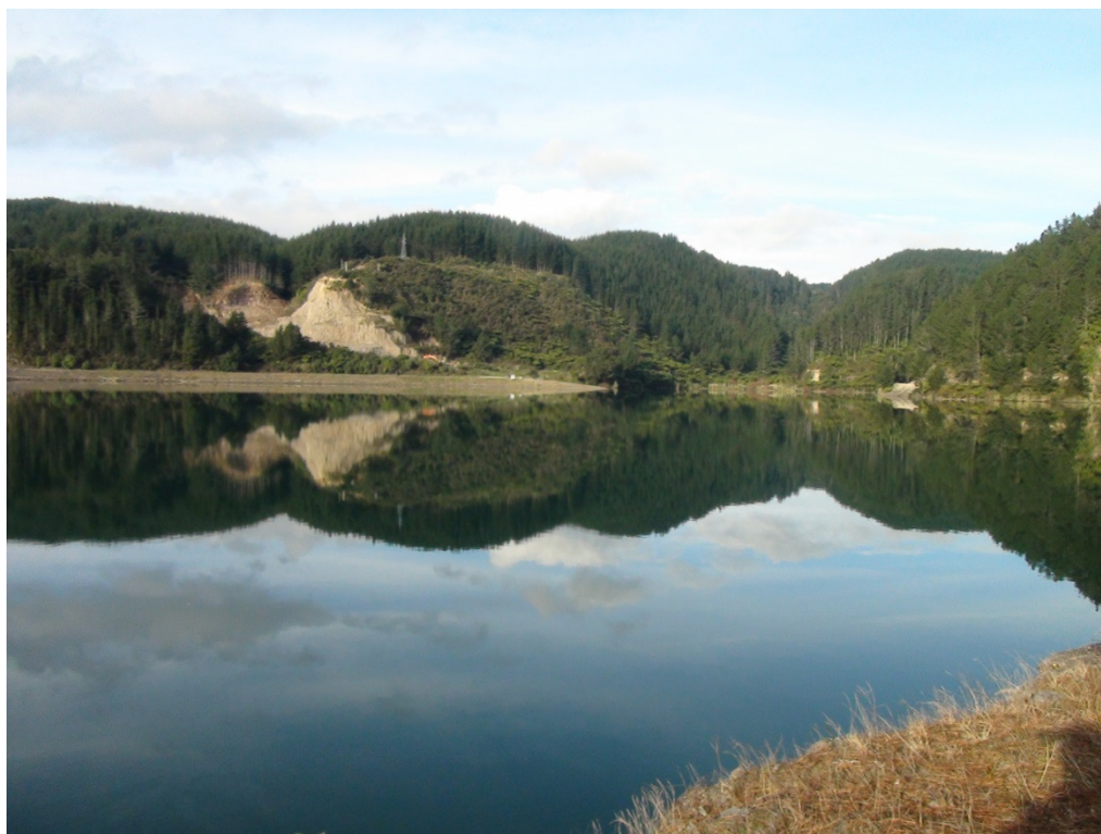
Rangitāiki River hydro dam and exotic forestry
