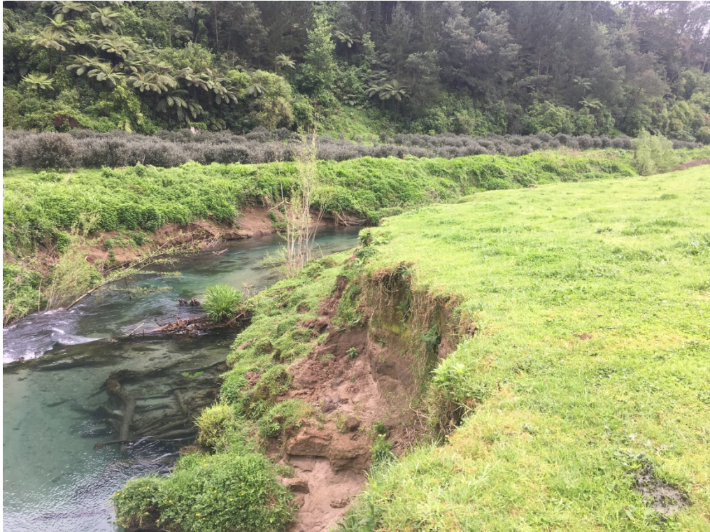
Streambank erosion on the Waiari Stream
