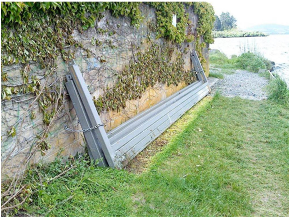
Figure 10 Ohau Channel stoplogs stored on site following refurbishment. Each stoplog is 6 m long x 0.3 m high.
