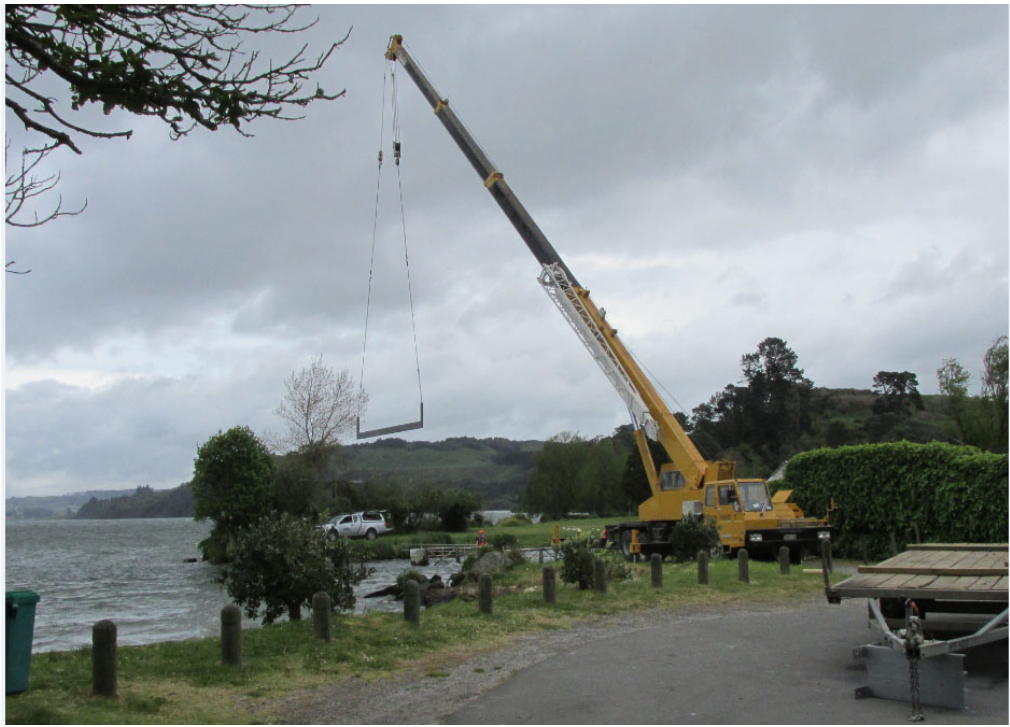
Figure 9 Installing Ōhau Weir stoplogs - 22 October 2015.
