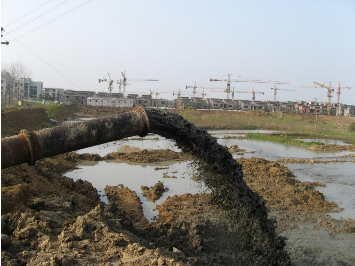
Figure 8. Dealing with dredged spoil can be a major operational issue and expense; a lake dredging operation in China.
