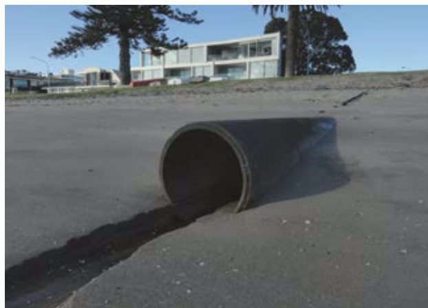
Figure 1: A stormwater outlet from an urban area. Sediment contamination is generally higher close to stormwater outlets.
