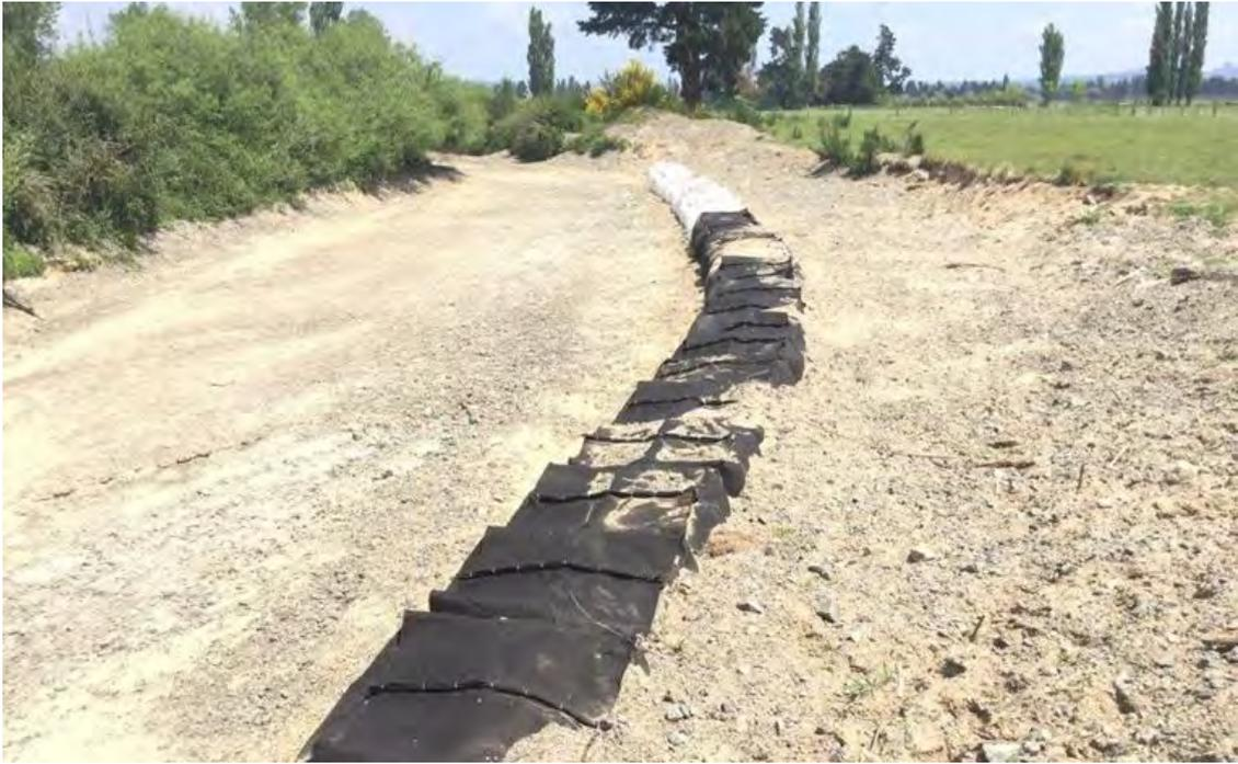
*Figure 6: Erosion repair using geotextile gabions, Mangamate Stream*
