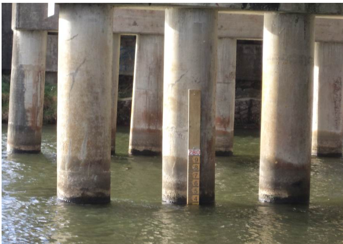
Figure 20 Ohau Channel Staff Gauge on State Highway 33 Bridge – Mourea.
