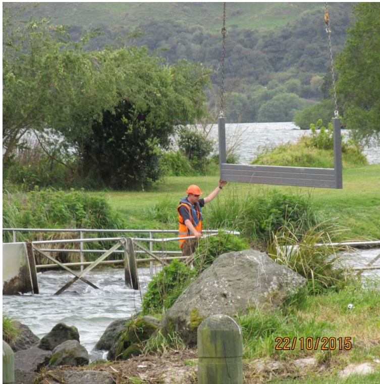
Figure 9 Installing Ōhau Weir stoplogs - 22 October 2015.
