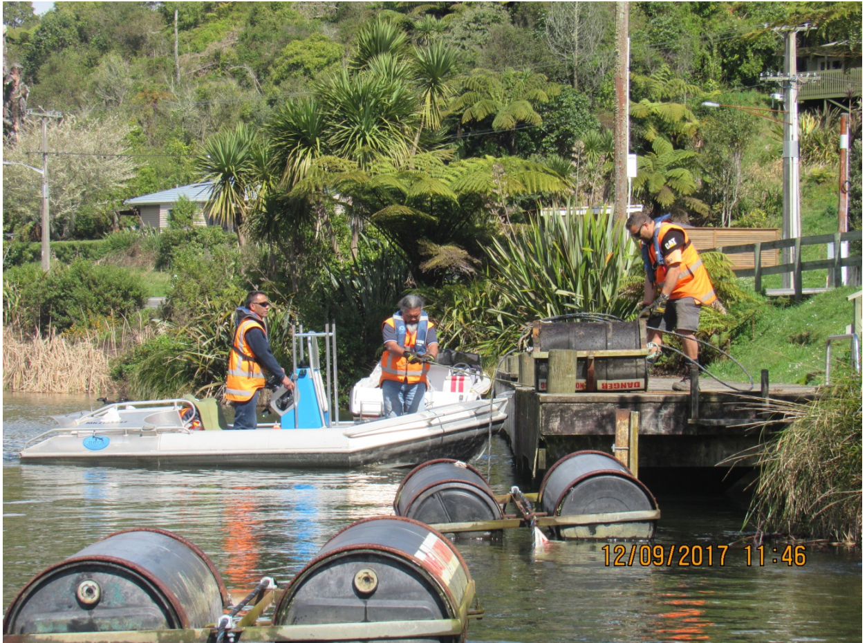
Figure 1 Okere Gates Barrage – Regional Council staff replacing barrage main line after failing in high flows – September 2017.
