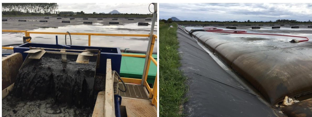
Figure 6. Contaminated sediment comes onto shakers, through the water treatment area and into the geobags.
