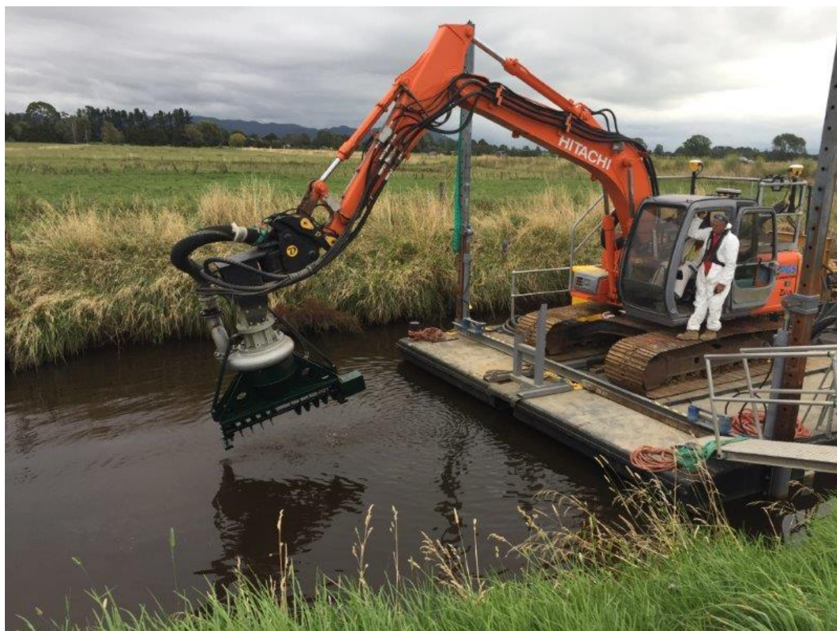
Figure 5. Dredging using auger cutter suction dredge head.
