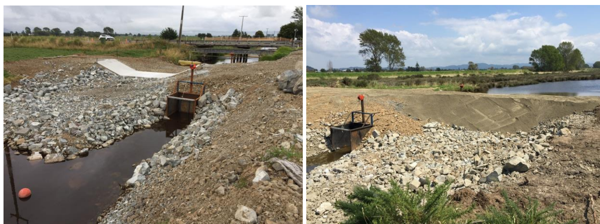
Figure 2. Kopeoepo flood control structures showing culvert, emergency spillway and sand plug.
