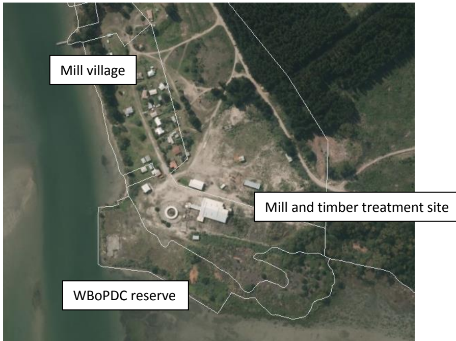
Figure 1: Matakana Island saw mill including the mill village and Western Bay of Plenty District Council reserve.
