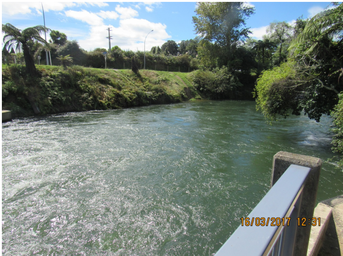
Figure 15 Kaituna River below Okere Gates – 3 gates @700 or 31 cumecs on 16 March 2017.
