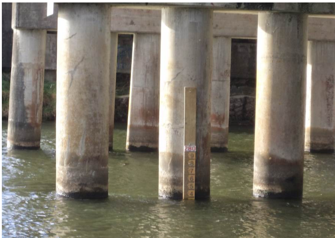
Figure 18 Ōhau Channel Staff Gauge on State Highway 33 Bridge – Mourea.
