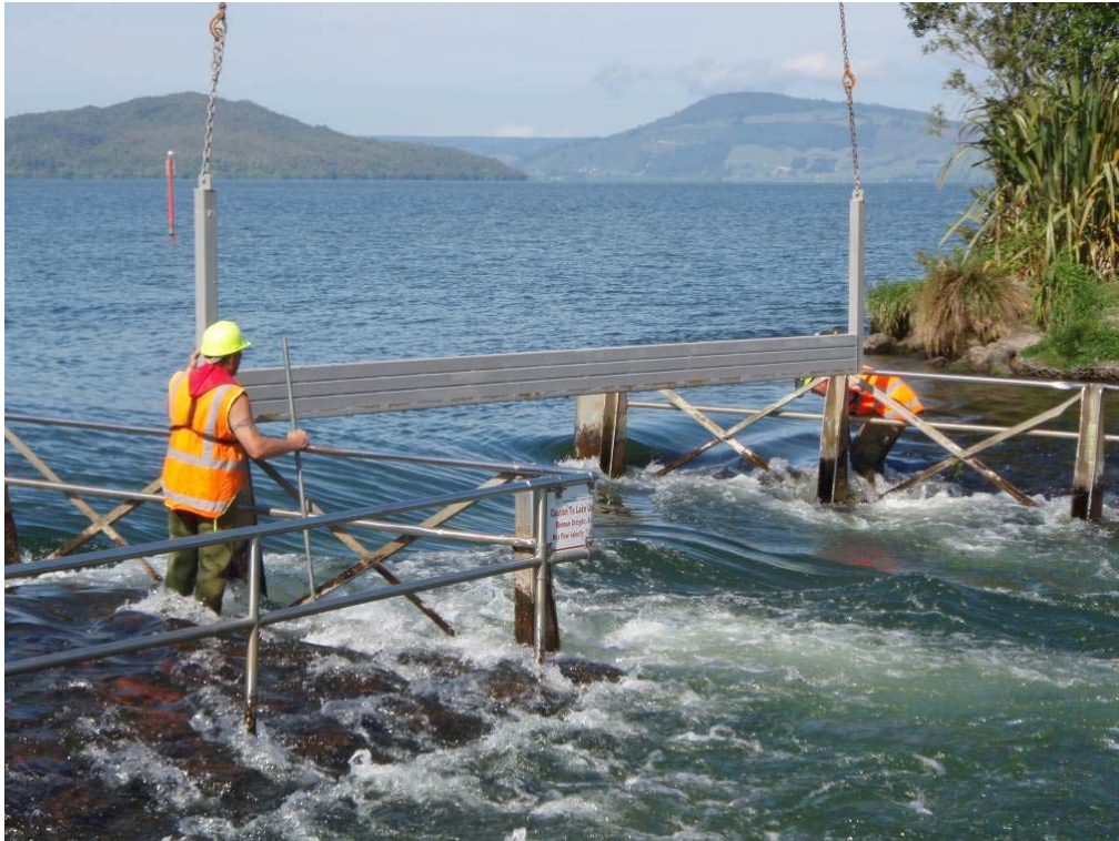
Figure 10 Removing Ōhau Weir stoplogs - 29 October 2010.
