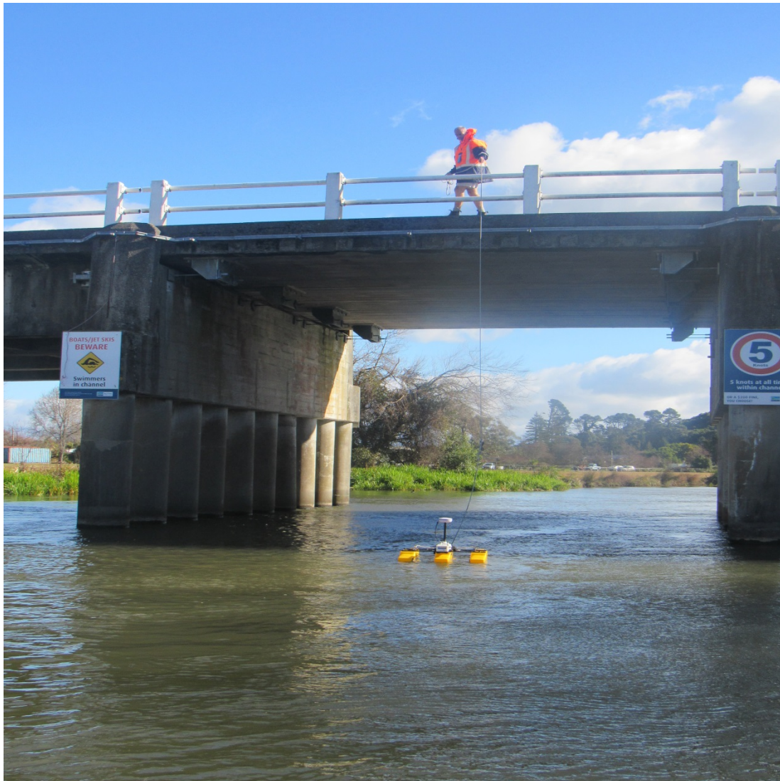
Figure 1 Ohau Channel at State Highway 33 Bridge – Regional Council staff measuring flow and velocity during annual drawdown of Lake Rotoiti – 20 July 2016.
