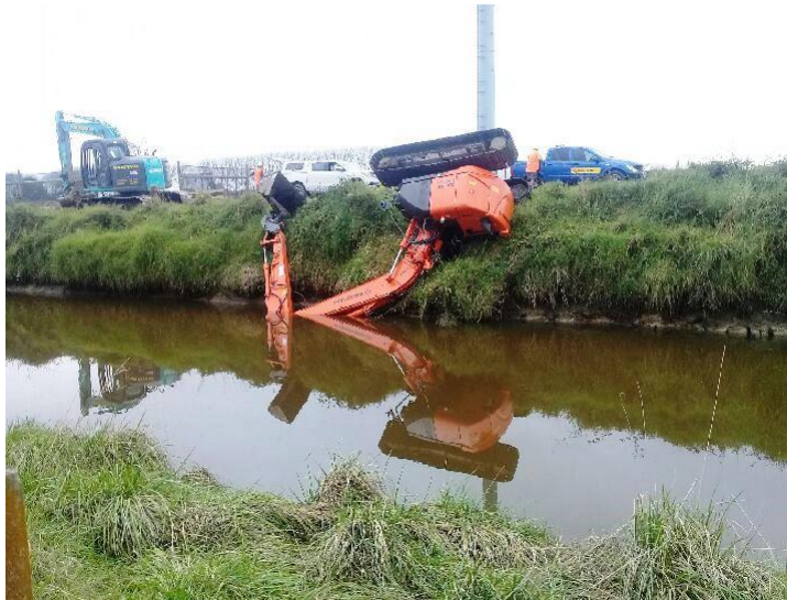
Photo 1 Notifiable Event: Excavator
