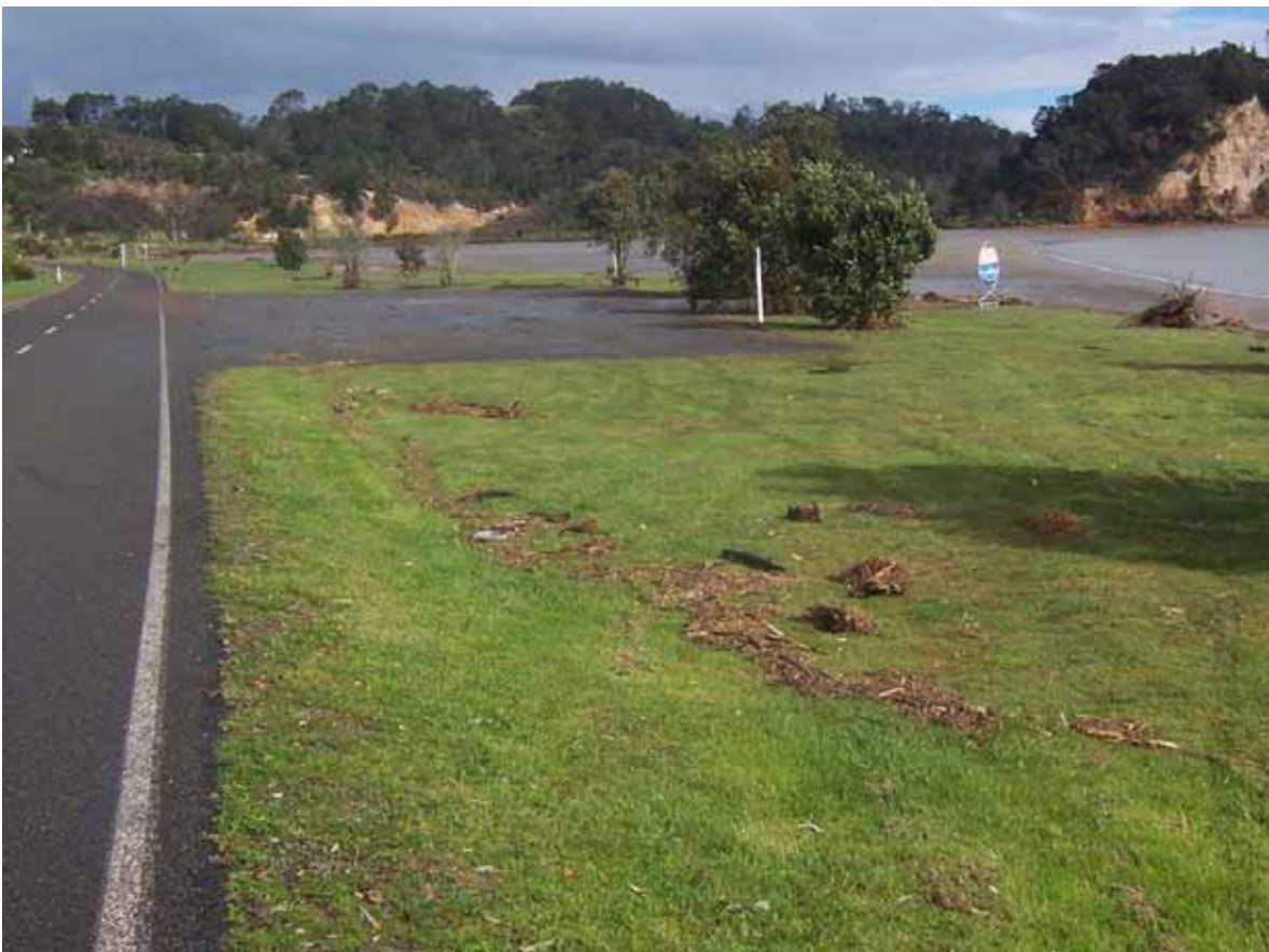
Boat Ramp, Ohiwa Loop Road
