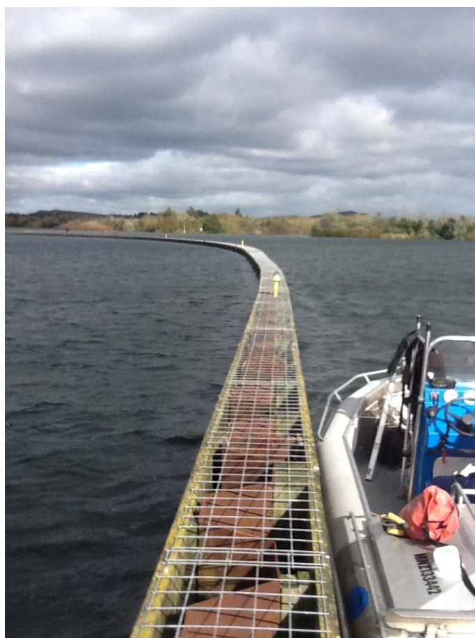
Figure 17 Ohau Diversion Wall – Annual inspection – 18 May 2015.
