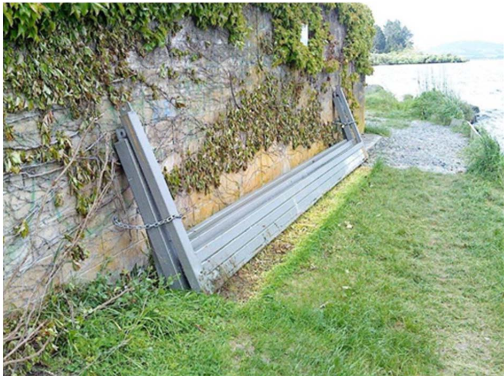
Figure 11 Ohau Channel stoplogs stored on site following refurbishment.
