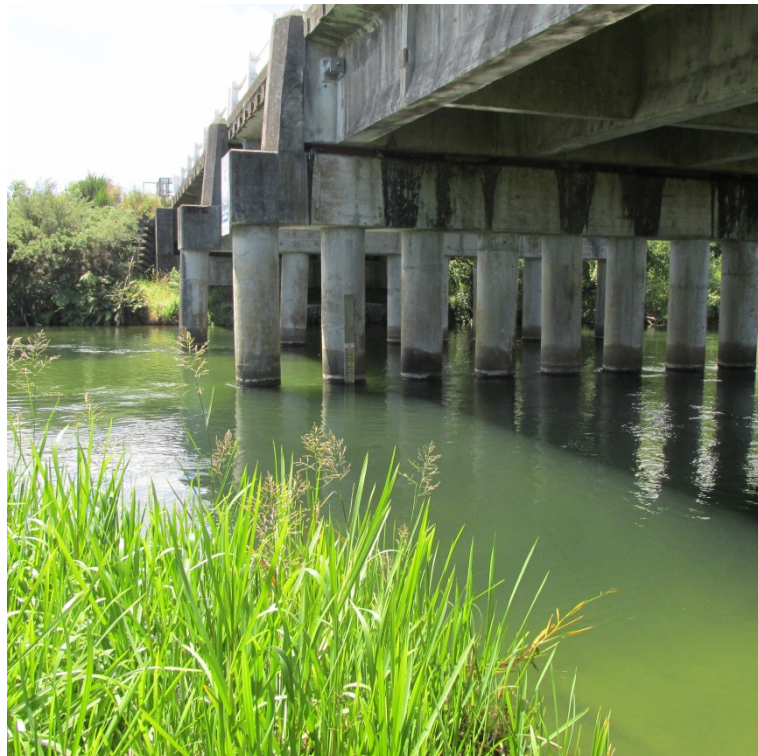
Figure 20 Ōhau Channel Staff Gauge on State Highway 33 Bridge – Mourea.
