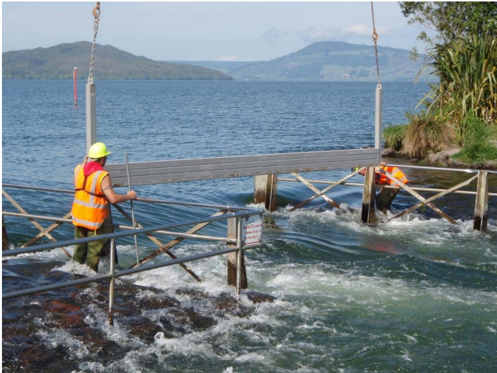
Figure 10 Removing Ōhau Weir stoplogs - 29 October 2010.
