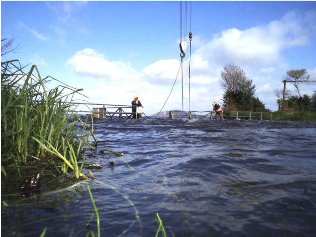
Figure 4 Removing Ōhau Weir stop logs - 27 May 2013.
