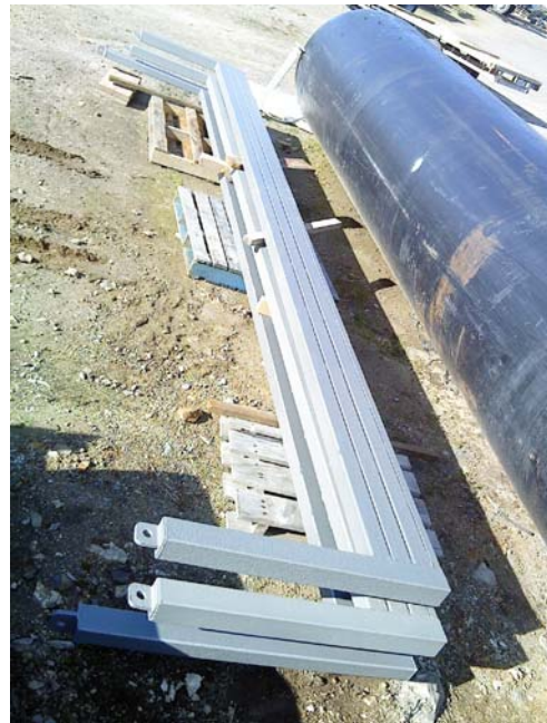
Figures 5 & 6 Following removal, the stop logs were found to be corroded and encrusted with barnacle growth prompting early maintenance to clean, repaint and replace all fittings.
