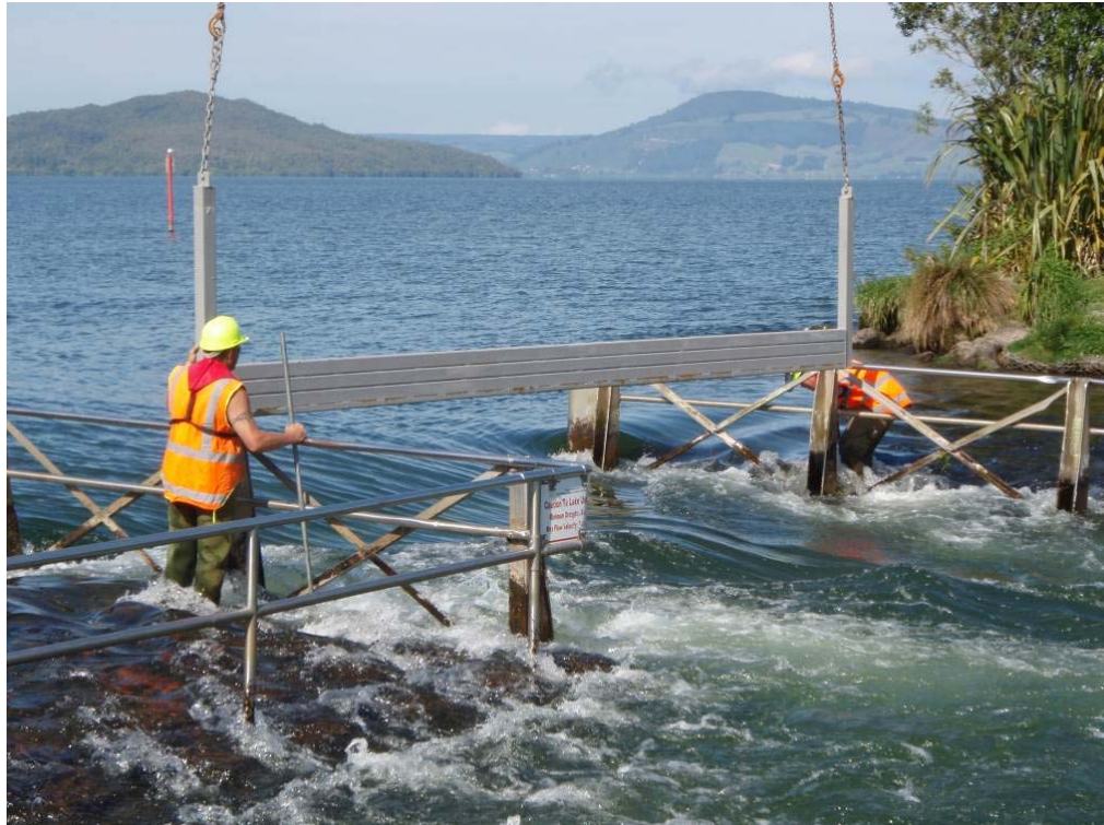
Figure 10 Removing Ōhau Weir stoplogs - 29 October 2010.
