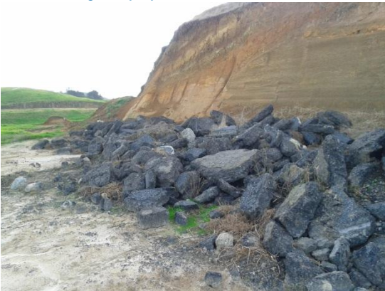
Figure 51 Demolition waste stored away from operational areas
