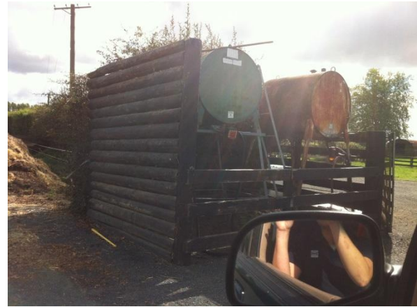
Figure 56 Confined storage of petrol and diesel tanks
