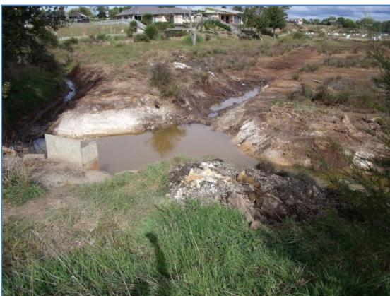
Figure 5 Downstream culvert on wetland side of stopbank.
