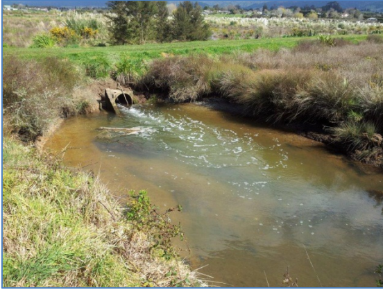
Figure 3 Downstream culvert on stream side of stopbank.
