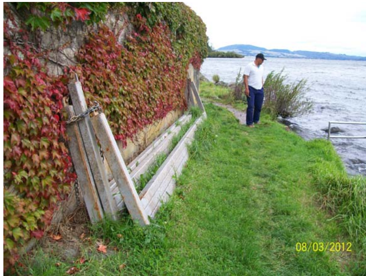
Figure 4 Ōhau Weir Stop logs (x3) stored onsite after removal (dimensions 6m x 0.3 m).
