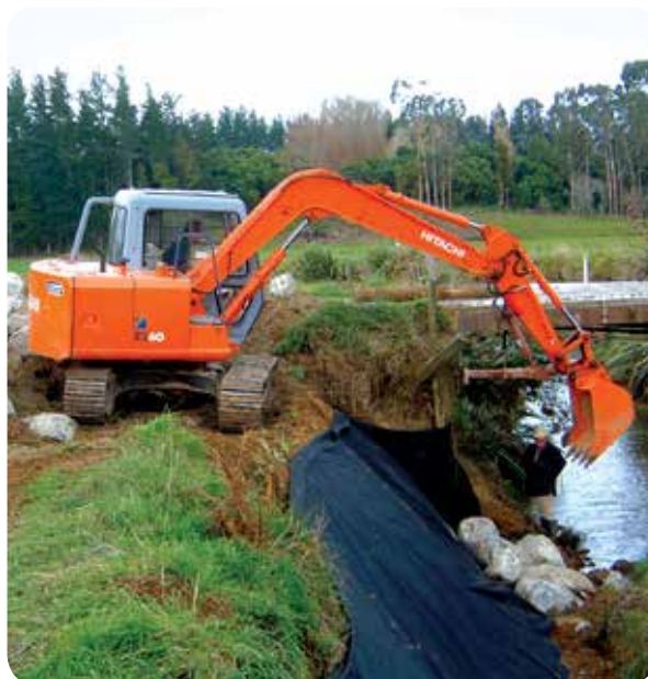
Photo: Constructing rock structure to protect farm bridge access.
