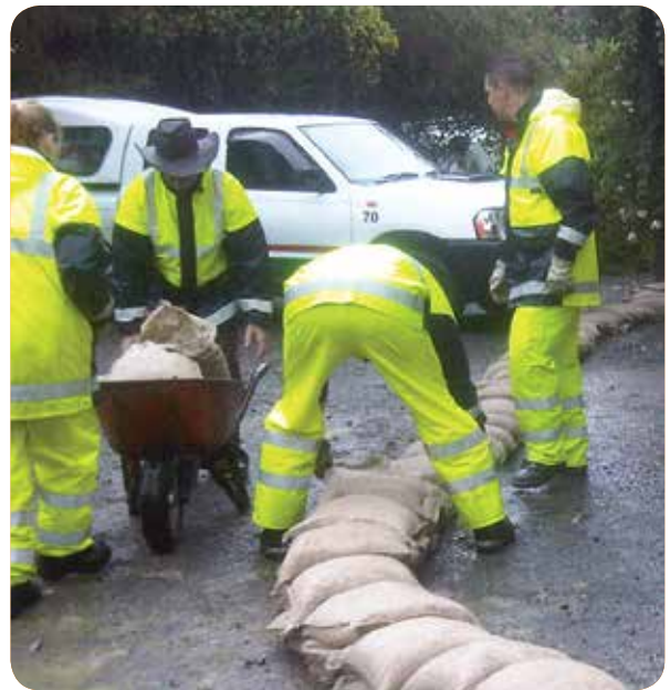
Photo: Bay of Plenty Civil Defence team preparing for flooding.
