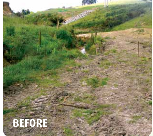
Photo: Riparian work retirement before and recently completed.
