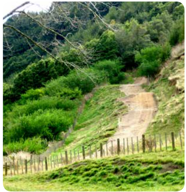
Photo: A farm track with humped water control cut-offs to divert flow off the track to grassed areas.
