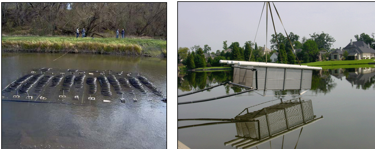
Figure 17 Closed water loops using HDPE pipes or a stainless steel plate heat exchanger.
