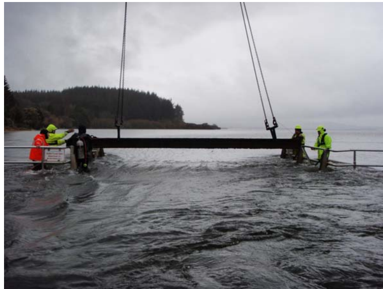
Figure 5 Ohau Weir Stop log removal in progress (12 August 2008).
