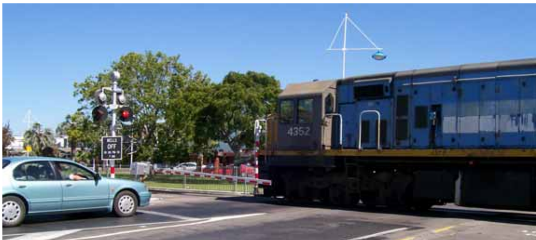
A second Tauranga Harbour Rail Bridge is a potential future project to address freight rail issues in the Tauranga CBD
